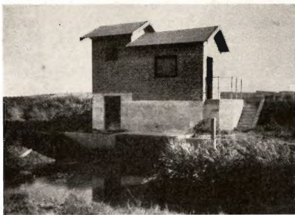
Tjæreby-Vestrup. Ny Pumpestation.
